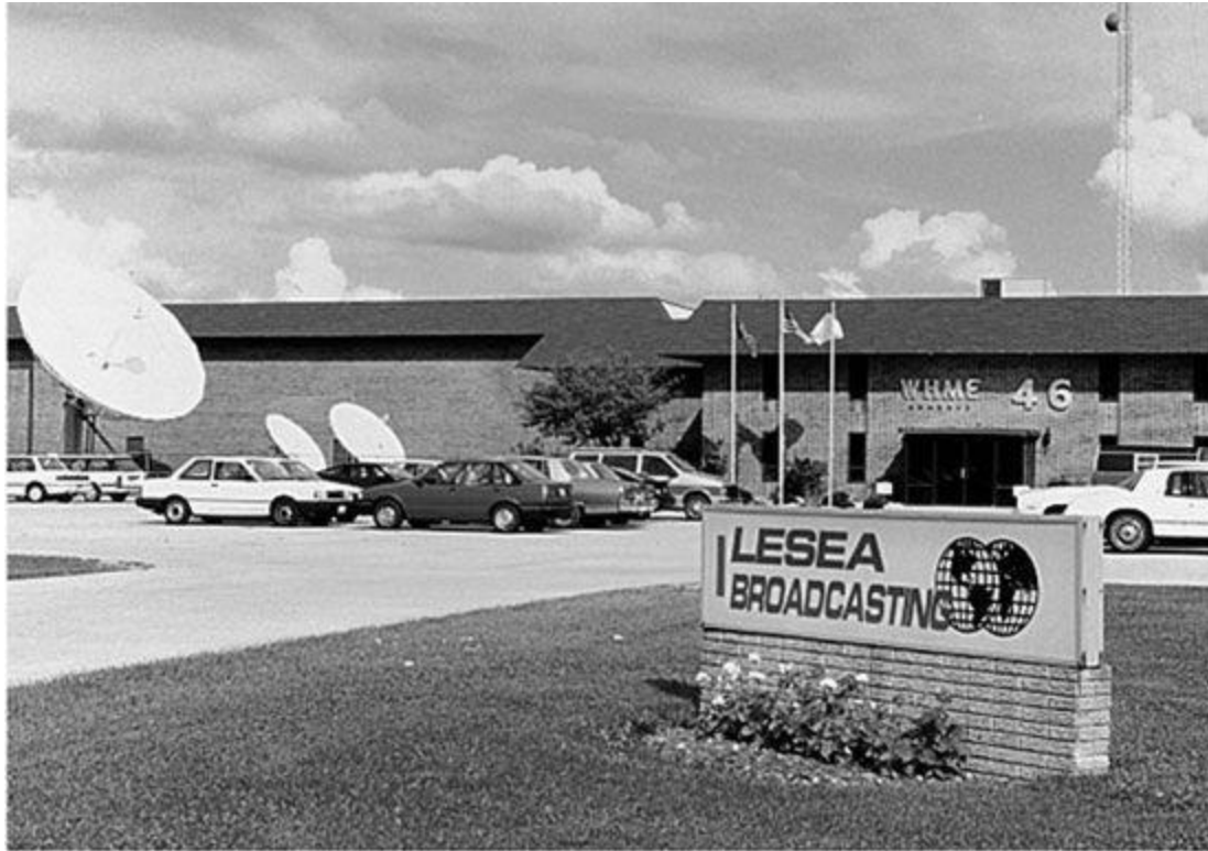
The reconstruction and renovation were completed in 1989.
